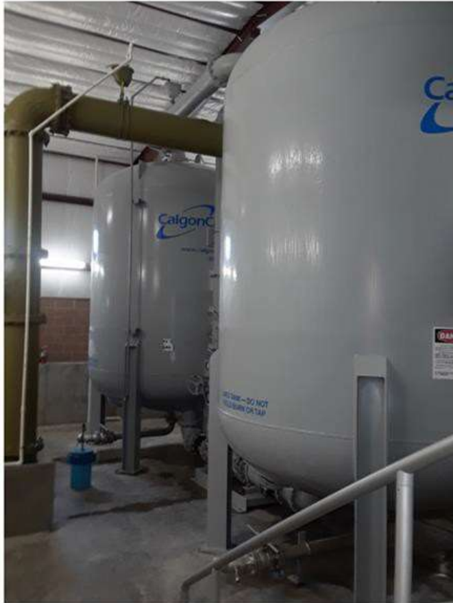
Vessels in place at the Southmoor Water Treatment Facility
