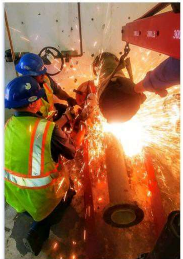
Water Operators Cutting Ductile Iron
